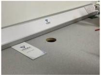
Using the hole cutter or similar, cut the hole through the bench—do not press to hard and overheat the cutter—take your time or it may burn or scorch the wood.
