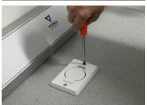
Locate the Flip Top assembly into the hole (see bottom image) - and fix with two self tapping or wood screws.
