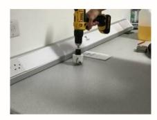
Decide and mark the hole position. Tip: Hold the arm/nozzle where you want it to be used and use this as a position guide. CHECK under the bench to ensure no framework is in the way!
